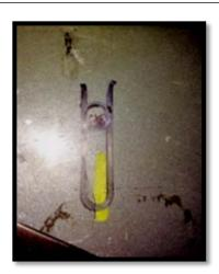
**Step 6:** Remove clip. Use a ½" drill bit and drill out the center mark. Slide the 3/8 clip back into position so the threaded part is aligned with the hole.
