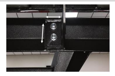
Step 7: After finial adjustment, torque each bolt to 17 ft/lb – 20 ft/lb.
