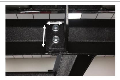
**Step. 8:** After finial positioning, completely tighten all (x6)  $\frac{1}{4}$ "-20 x  $\frac{3}{4}$ " in the pinch weld attachment.
